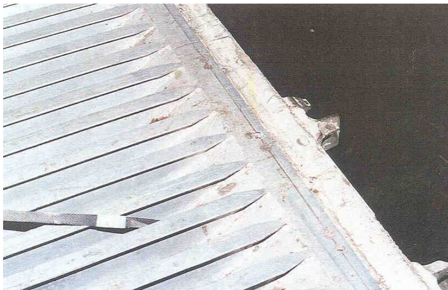
Entrance to container, T-grating floor screwed in place.
